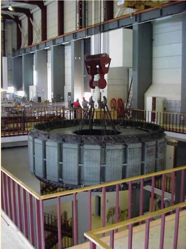
■ FIGURE 12.21 The 24-pole rotor of a synchronous generator as it is being lowered into position. (Photo courtesy Dr. Wade Enright, Te Kura Pukaha Vira O Te Whare Wananga O Waitaha, Aotearoa.)
