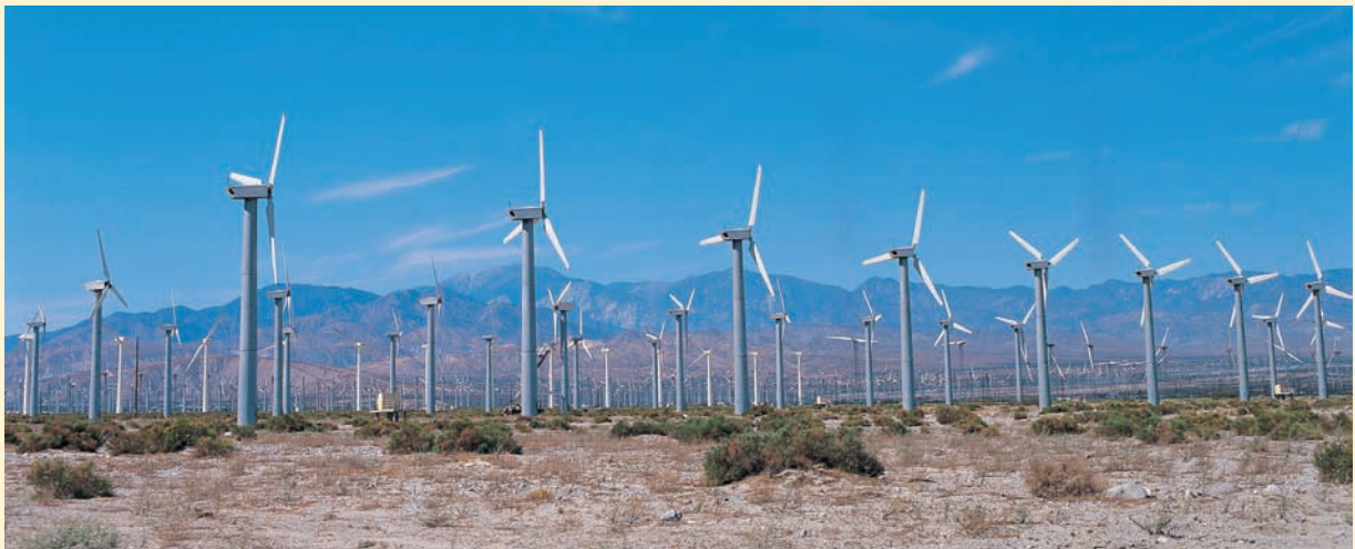
■ FIGURE 12.20 Wind-energy harvesting installation at Altamont Pass, California, which consists of over 7000 individual windmills. (© Digital Vision/PunchStock)
