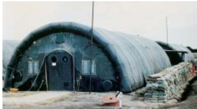
Fig. 6-4. An inflatable shelter in use in Vietnam, 1967. The MUST (medical unit, self-contained, transportable) surgical hospital used two characteristic structures: hard-walled, expandable shelters that contained the operating rooms and supporting services; and inflatable shelters that served as patient wards. Although representing an advanced-technology approach to providing a deployable surgical facility, inflatable shelters were probably not worth the effort. Setting them up was not easy and the equipment required to keep them inflated was labor-intensive. The inflatable shelters were also notably sensitive to battle damage.
